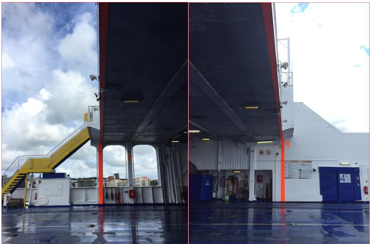
Figure 42: Left picture: Cargo RoPax bigger openings port side that needs to be closed. Right picture: starboard side at the same location
