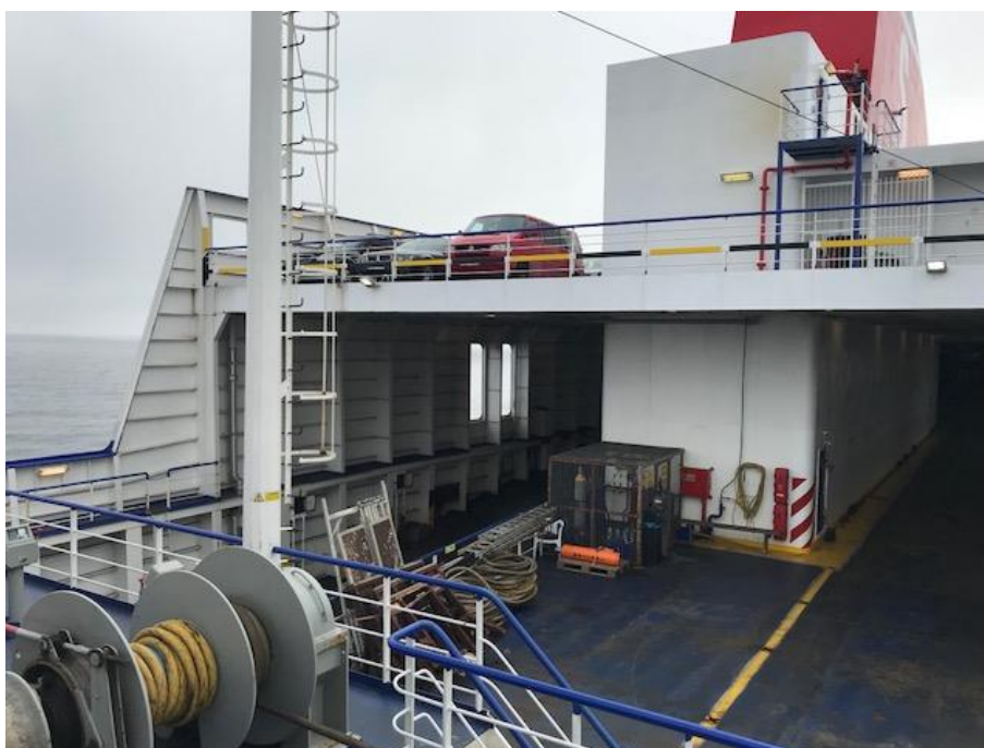
Figure 25: Picture illustrating a part of the aft opening on the Standard RoPax selected.
