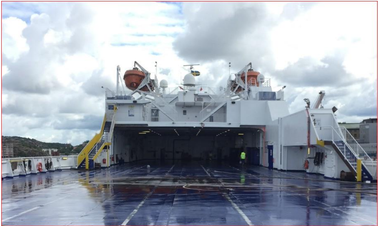
Figure 41: Cargo RoPax from the aft. Slight adjustments to the opening and the roll will be located just above the opening
