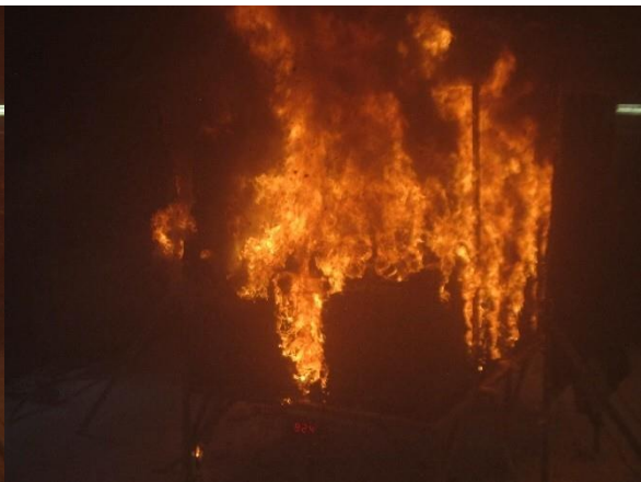
Six minutes after system activation.
