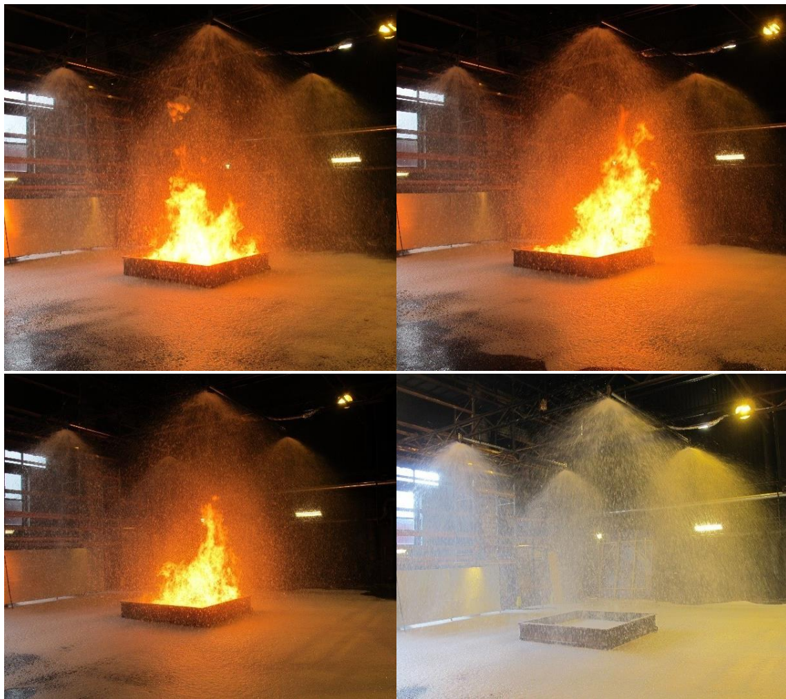
Figure 10: Fire testing in accordance with UL 162 of a foam-water spray system. A flammable liquid pool fire was extinguished within a few minutes. Photo: RISE.
