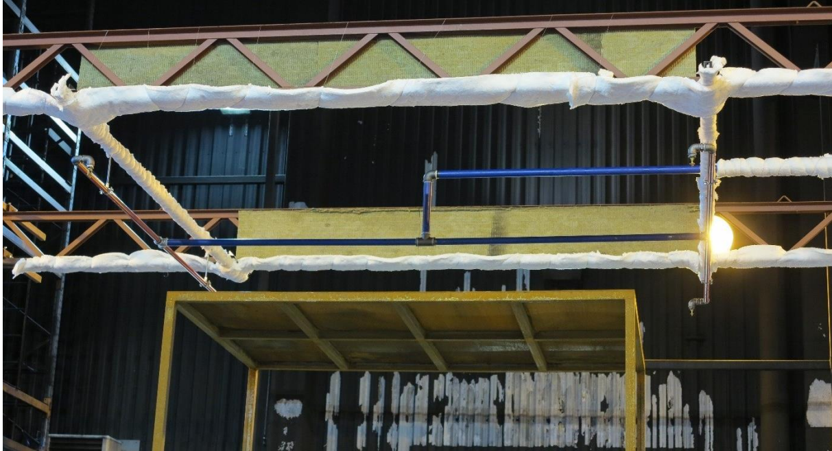
Figure A2-5: The pipe-work and its support beams. The support beams were insulated to protect them from thermal exposure
