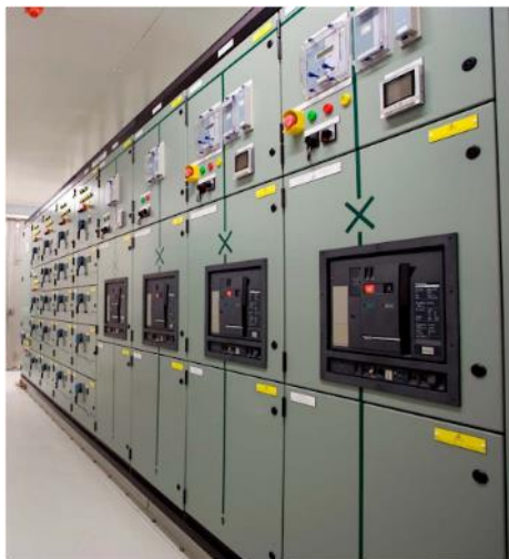
Figure 3.51 – Typical switchboard front panel view.
