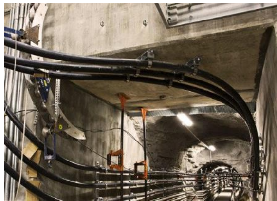
Figure 3.27 – HV cabling installation routed in tunnel.
