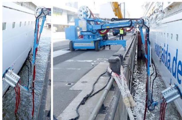
Figure 3.104 – OPS mobile CMS – compensation for tidal movement of the vessel is a fundamental functional role of all CMS equipment.
