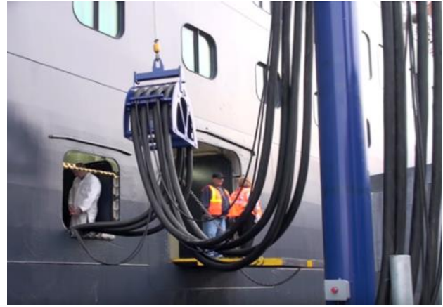
Figure 3.112 and Figure 3.113 – OPS fixed CMS – Port of San Diego – crane assisted handling of the HV feeders (including neutral and communications).
