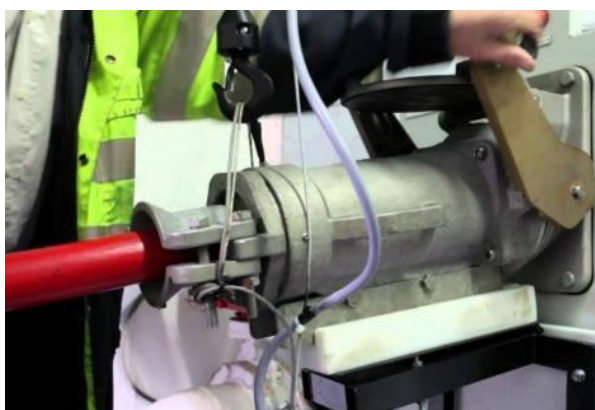
Figure 3.131 – HVSC plug and socket outlet - containerships.
