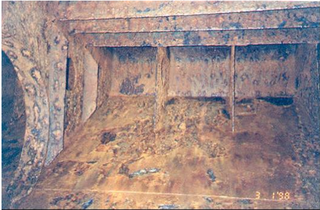
Poor paint application, ballast tank condition after 13 years (a bulk carrier top side tank is shown in this example)
