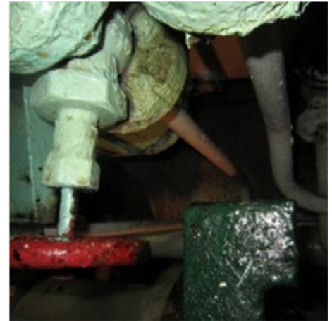
Bilge well (at the background)
