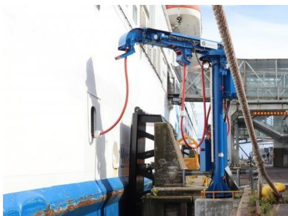
Figure 4.10 – OPS connection to RO-Pax ship.
